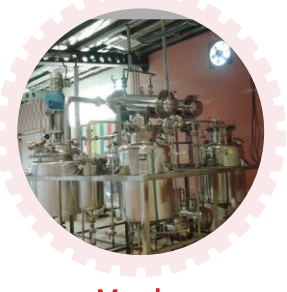
Myrrh Distillation Plant
